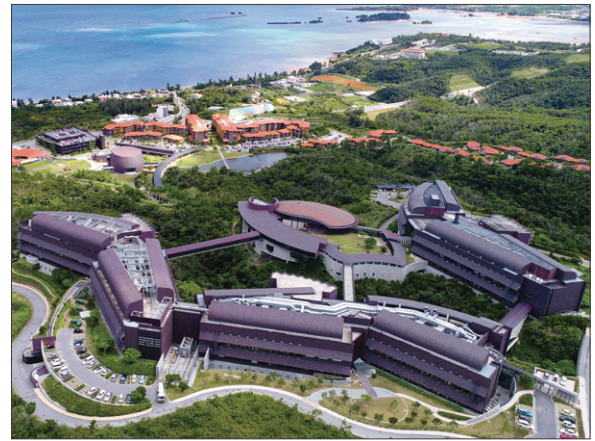
Figure 9-10 An aerial view of existing lab buildings
