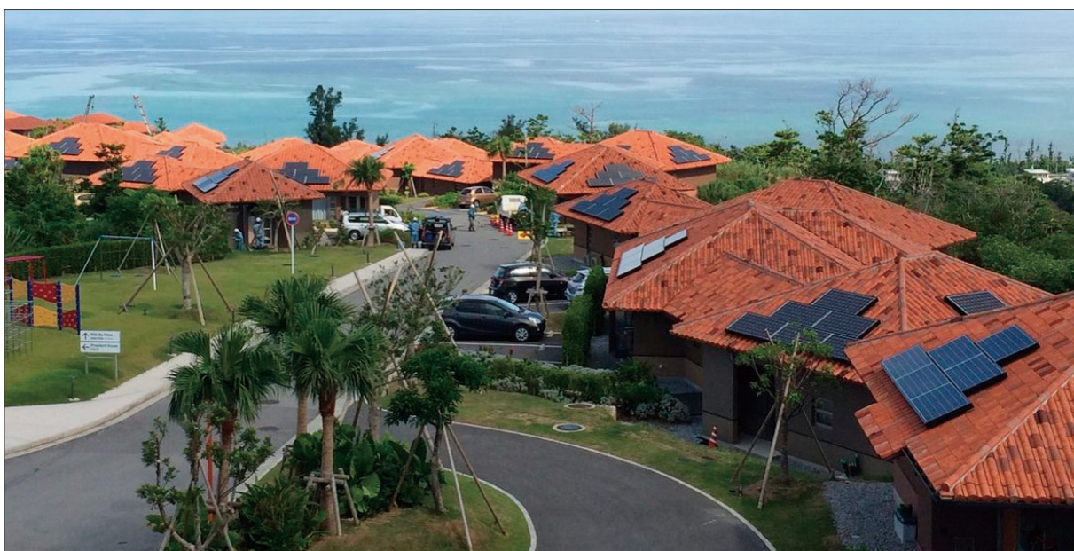
Figure D-5 Integrated open systems can support sustainable living and be built, for example, around artificial intelligence and the "internet of things". They can help to improve many areas impacting everyday life including the self-sufficiency of solar-powered houses connected on microgrids for energy transfer or battery management systems serving electric vehicles.
